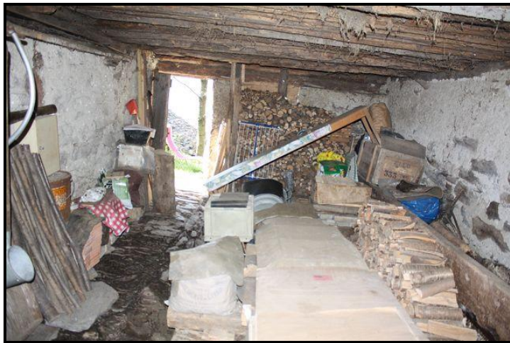
Locale PT / Erdgeschoss
